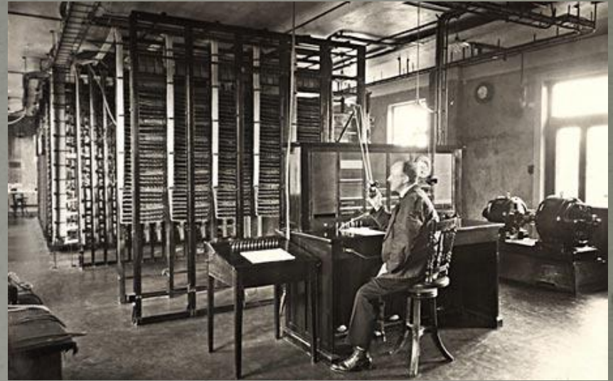
Automatic telephone exchange (~1910)
