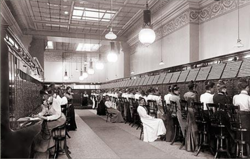
Manual telephone exchange (< 1900)
