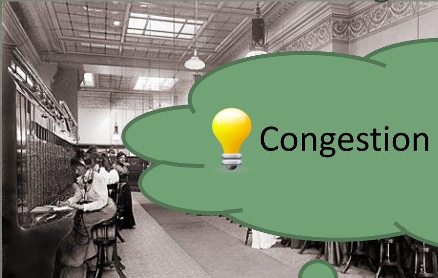
Manual telephone exchange (< 1900)
